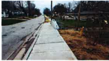
59th Street Culvert Improvements
