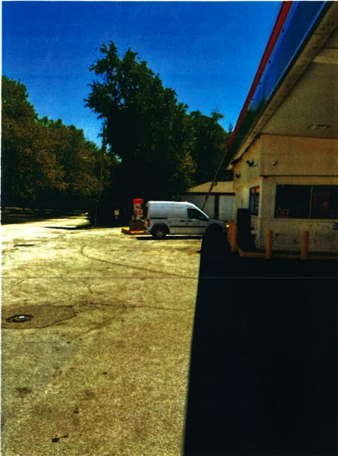
Figure 3: Zoomed out view of north side looking east showing open frontage onto 69 th Street
