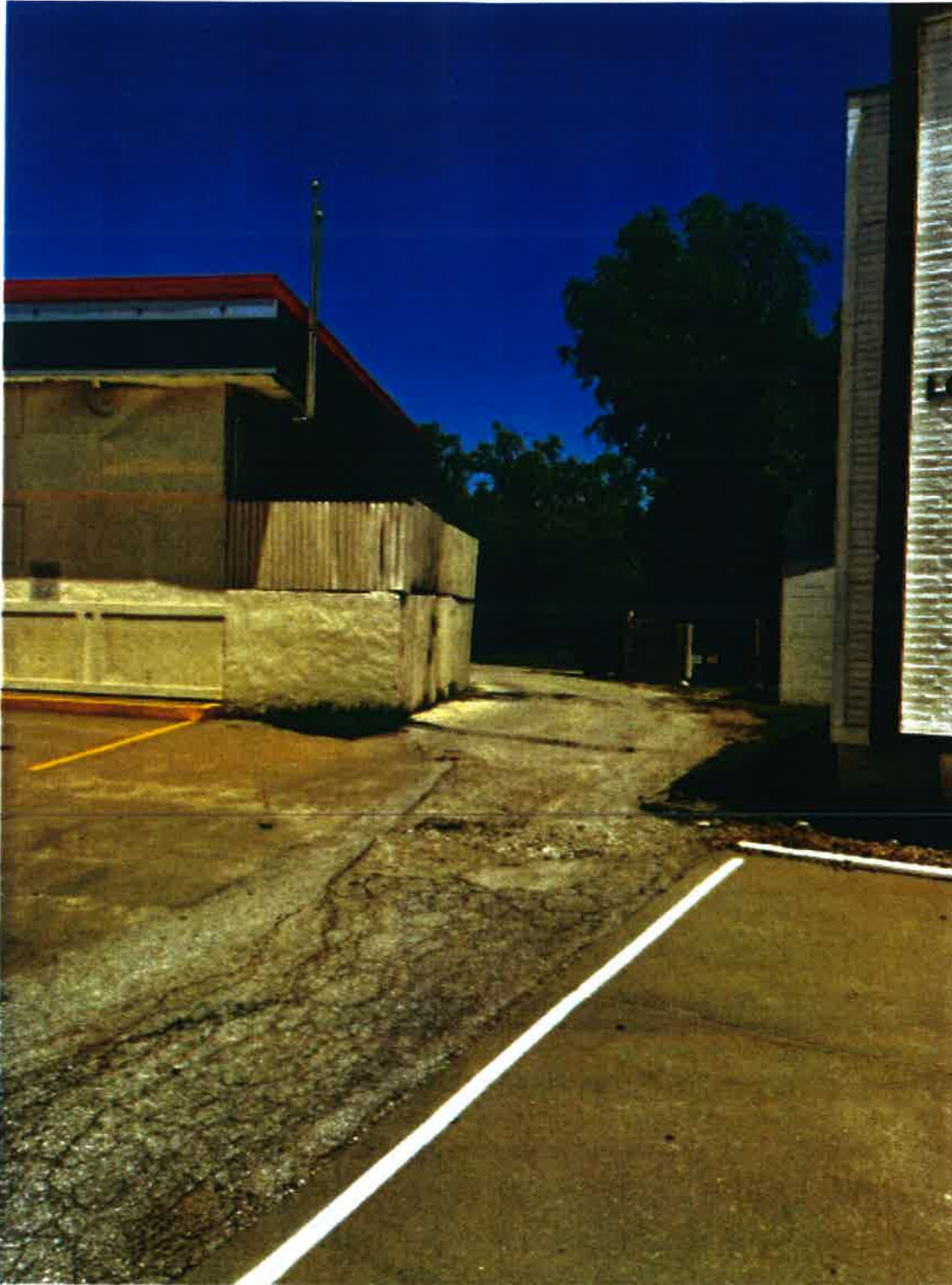
Figure 5: East side of building looking north toward 69 th Street showing fire access lane, dumpster enclosure and wall of adjacent Vet Clinic on right side of photo.
