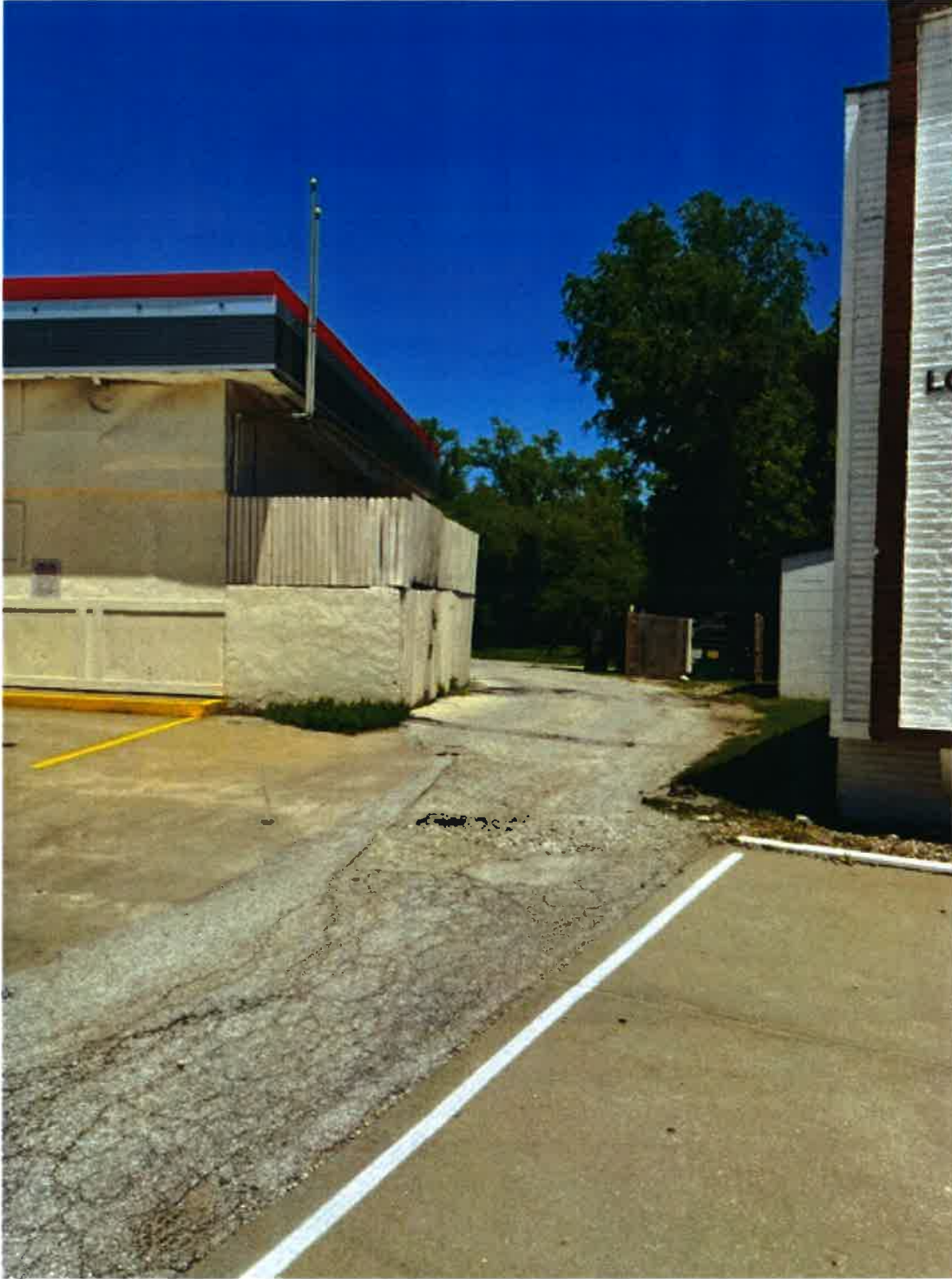
Figure 5: East side of building looking north toward 69 th Street showing fire access lane, dumpster enclosure and wall of adjacent Vet Clinic on right side of photo.
